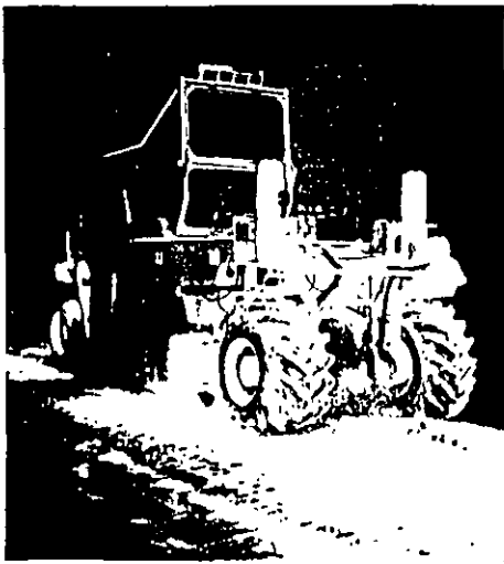
Wirtgen cold recycling: the existing road materials are reused to produce a strong foundation course.
