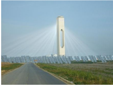
Figura 4.7. Central Solar Termoelectrica PS10
