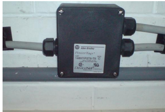
Figura 2.2. Power-Tap DeviceNet®.
