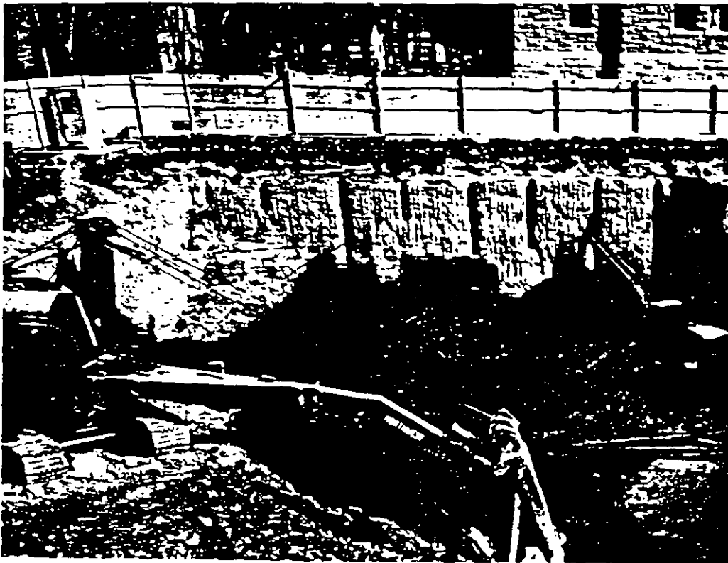
CUSHION BLAST RESULTS USING LARGE DIAMETER CUSHION HOLES AND SMALL DIAMETER GUIDE HOLES
