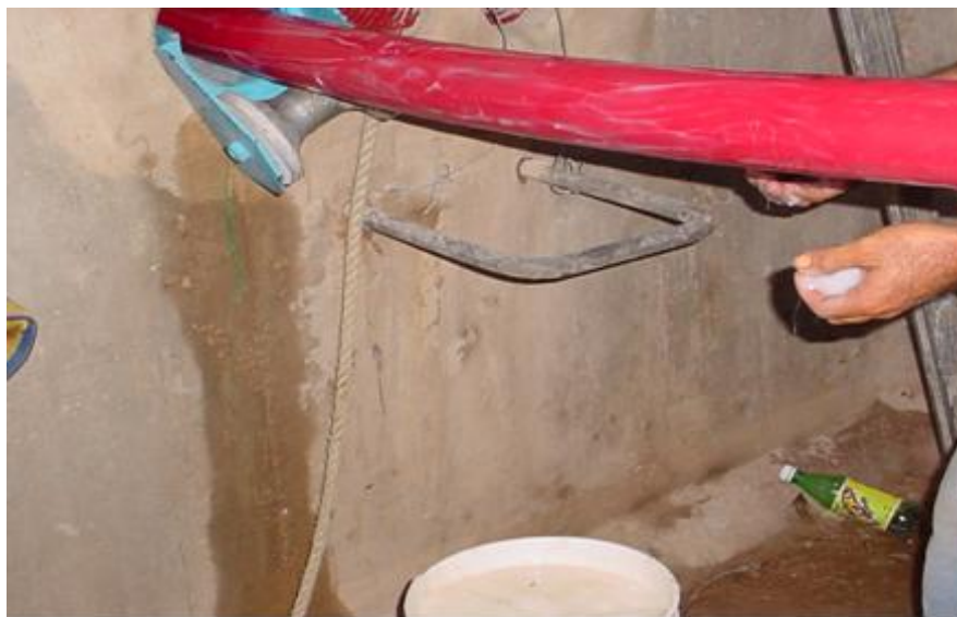
Figuras 1-11 Engrasado del conductor
