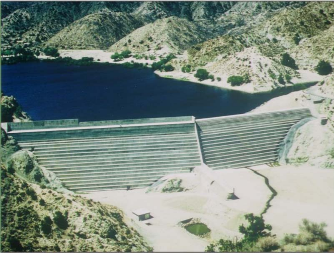
Figura 1- 24 Littlerock Dam California Rehabilitada con CCR (Hansen K. , Rehabilitation of Existing Dams with RCC, 2008)
