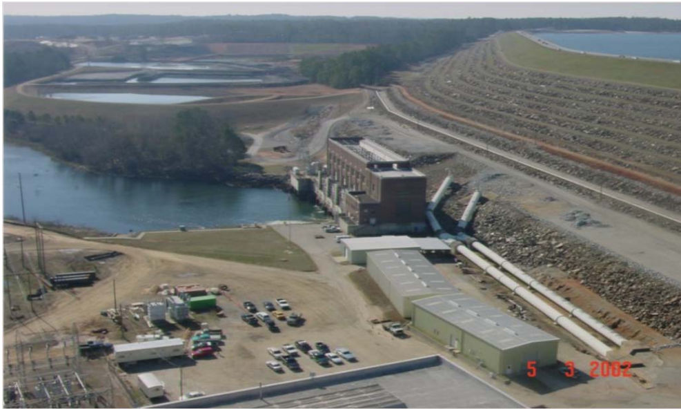
Figura 1- 26 Saluda Dam South Carolina, Usa (Rizzo C., 2008)
