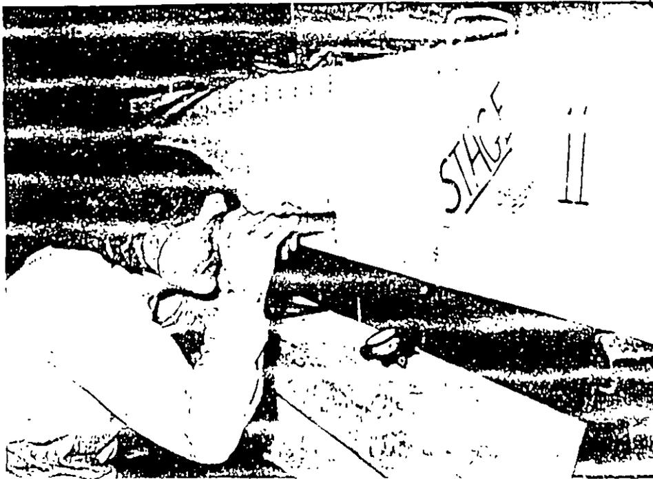
Photo 37 Simply supported beam prior to developing diagonal tension crack (load stage 11) (Test by Nally et al.)
