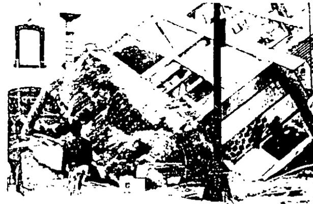
Fig. III-4.5: Collapse of a building on friction piles
