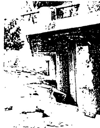
Fig. III-4.2: Earthquake induced tilt and settlement of a building on a mat foundation
