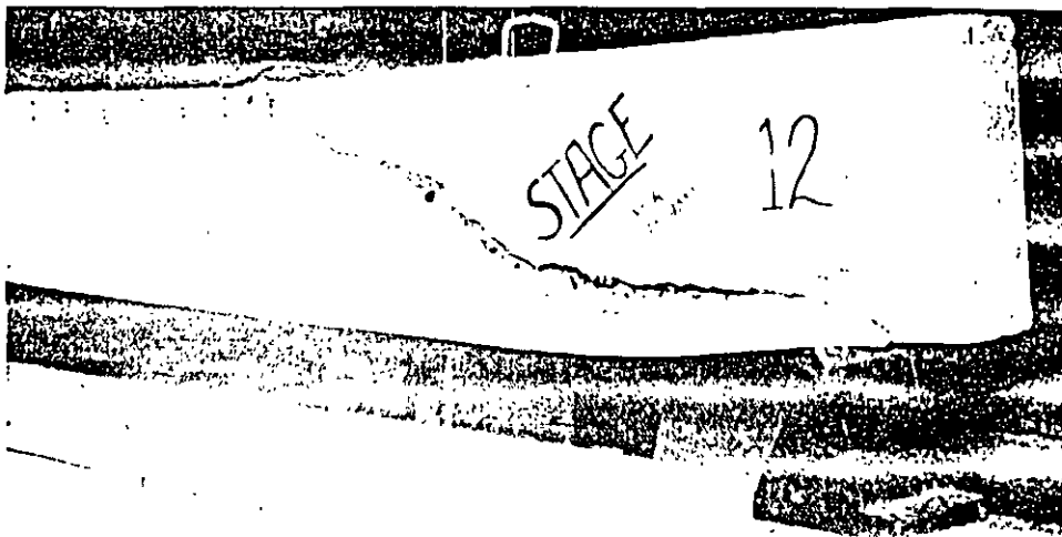
Photo 38 Principal diagonal tension crack at failure of beam in the preceding photograph (load stage 12).
