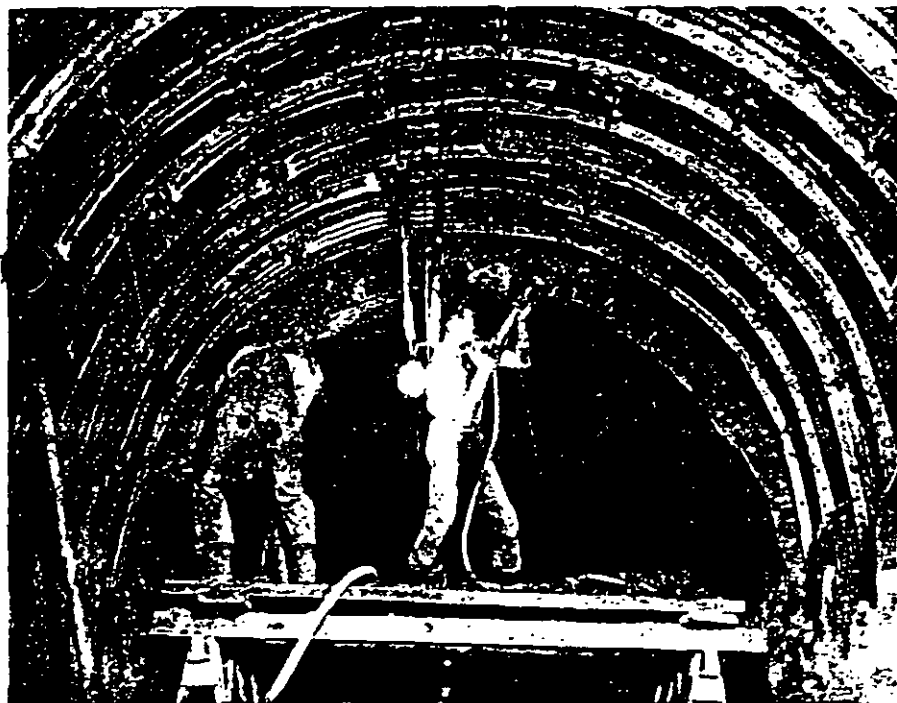
Fig. 44—Repair of damage to permanent tunnel lining in squeezing rock.
