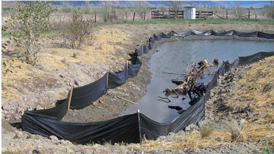
Figure 3.2 Wetland offsetting for Hwy 97 A new pond built by researchers from Ontario's University of Waterloo and the B.C. Transportation Ministry. Researchers hope amphibians that live in the area where Hwy. 97 is being expanded will colonize the new wetland area. Photo submitted.
