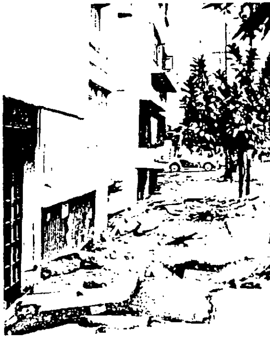
Figure 4 - Settlement of Building 1b.
