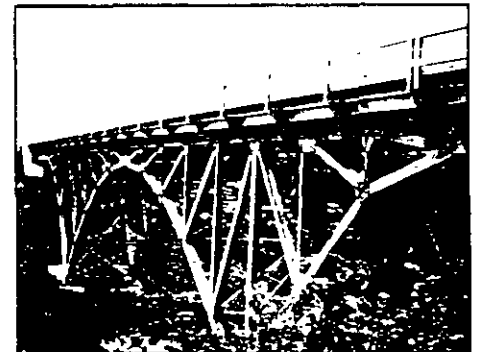
Fully Galvanized Lizotte Bridge
