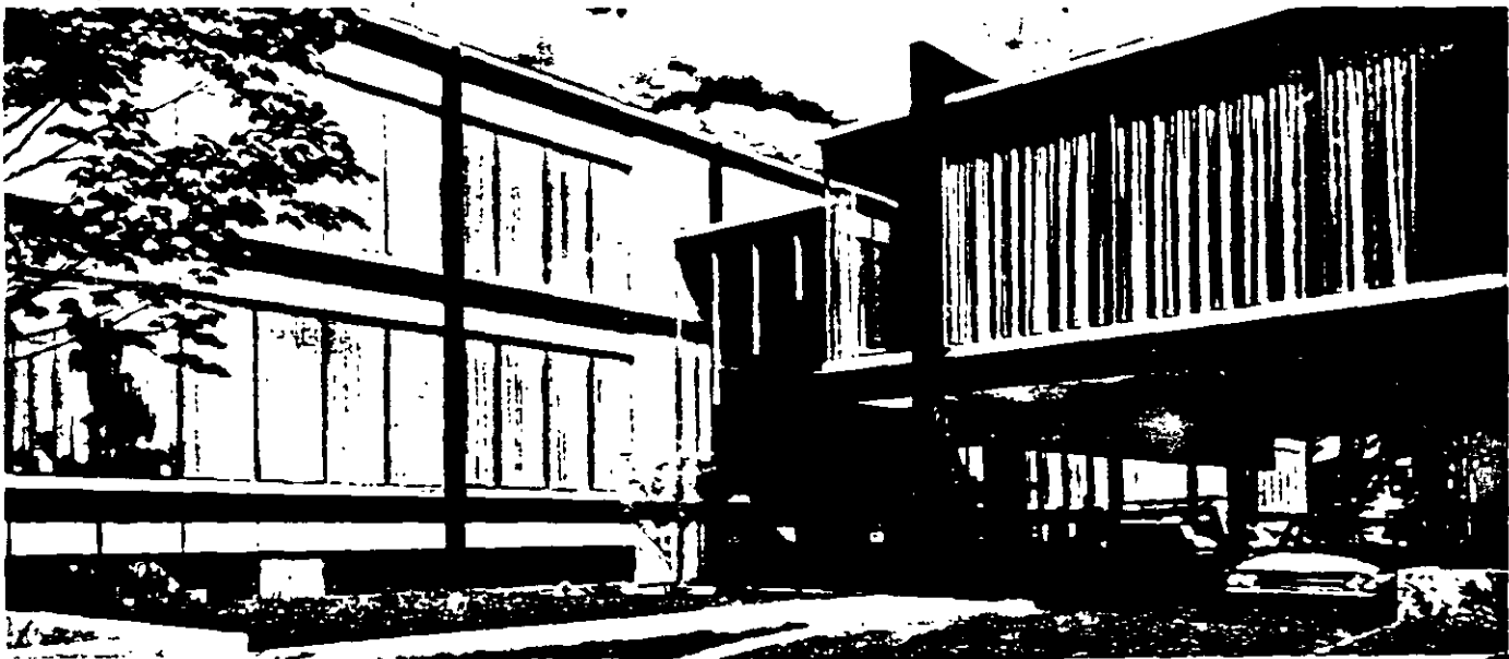
FIG. 8 Many contemporary structures are using exposed steel framing as part of the artistic scheme. Welding provides the unencumbered simplicity of form essential to the modern look in architecture, typified in this showcase building.
